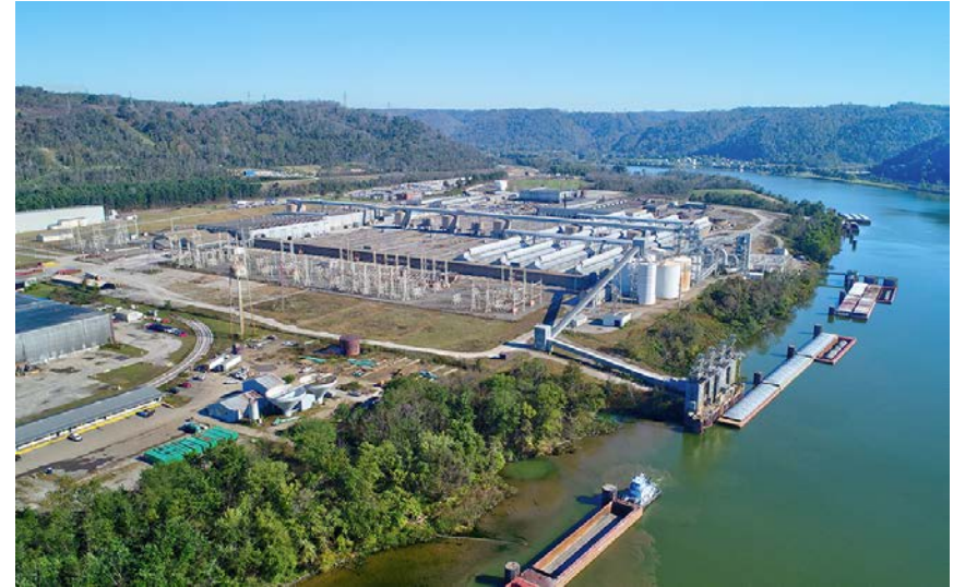
Long Ridge Energy Terminal
