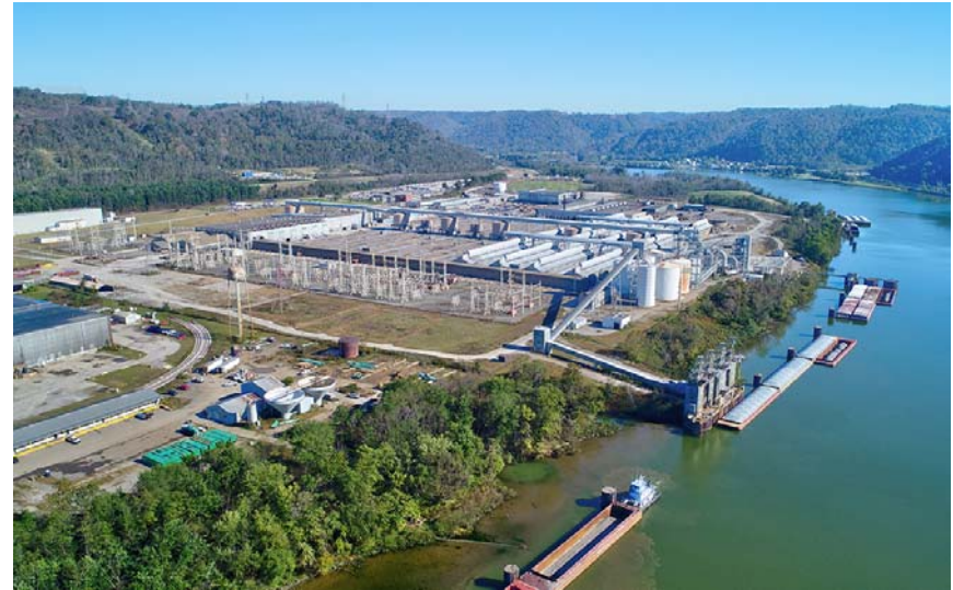
Long Ridge Energy Terminal
